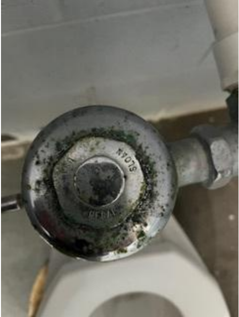
Fixed toilet at Sertoma.
