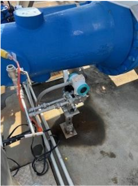
Replaced flow meter at water plant. John and Zane.
