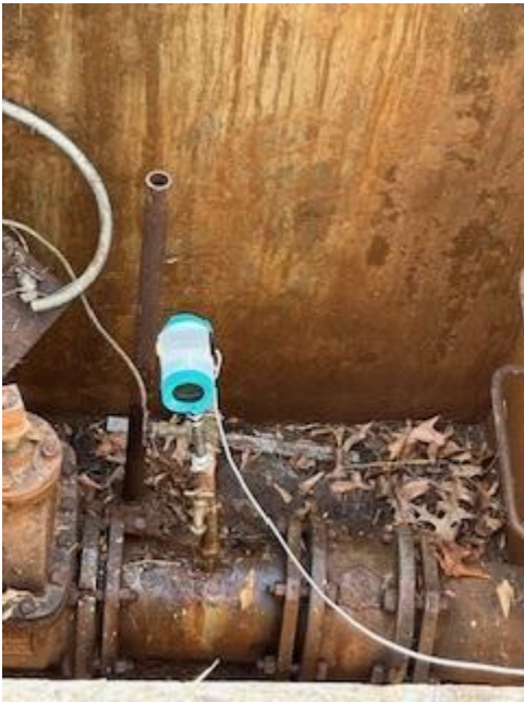
Changed pressure meter at water tank. John and Zane
