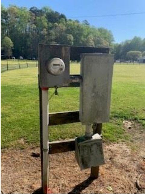
Fixed and secured Electrical box.
