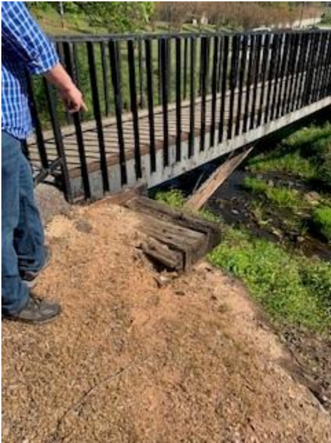
Hammered rebar in on bridge.
