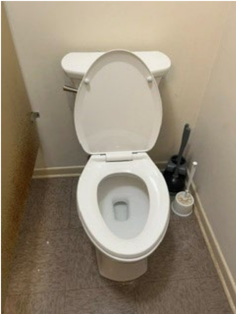
Replaced Depo Toilet.
