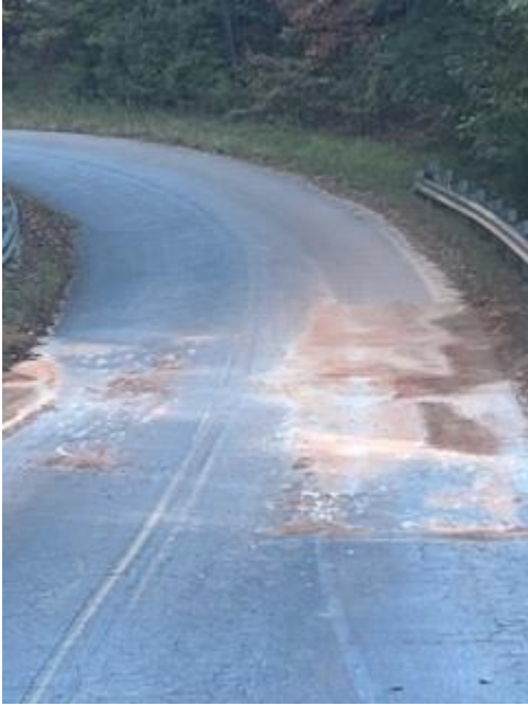
Cleared Woodland way of grave and dirt.
