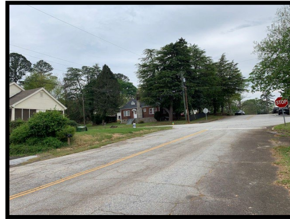
Looking West along Booker Drive (Intersection of Booker Drive and South Tugaloo Street)
