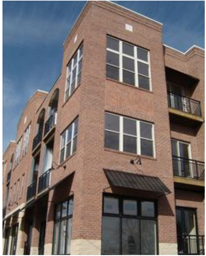
Example of compatible modern construction
