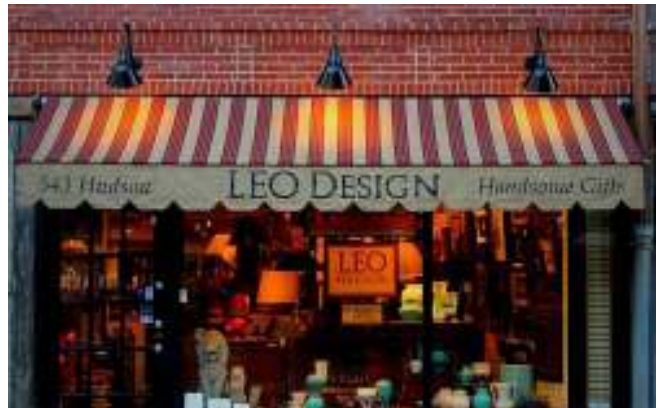
Lighting attached to facade illuminating canopy
