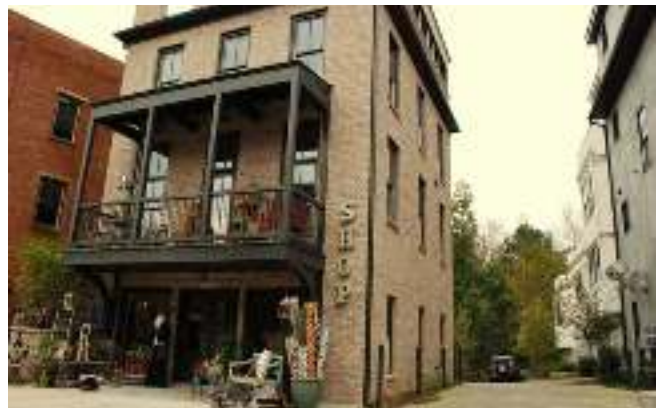
Example of compatible modern construction
