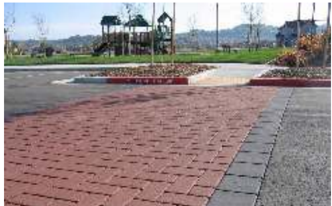
Example of decorative intersection paving
