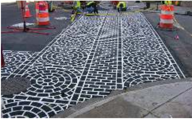
Example of decorative intersection paving
