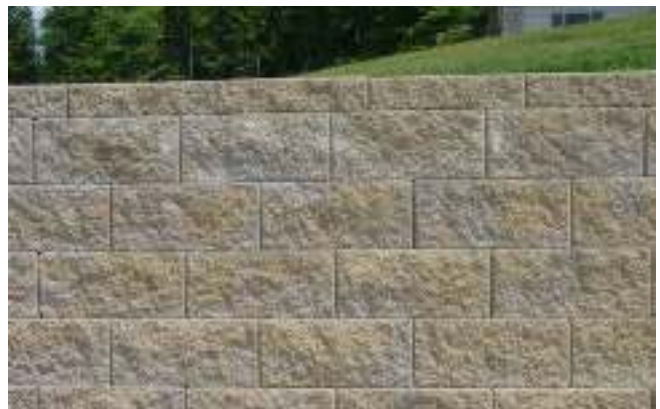
Example of split-faced masonry wall
