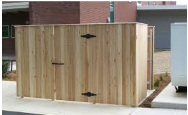
Example of mechanical enclosure
