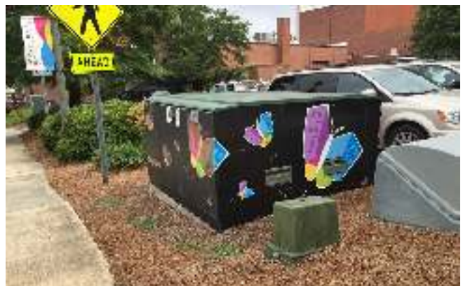
Example of trash storage area
