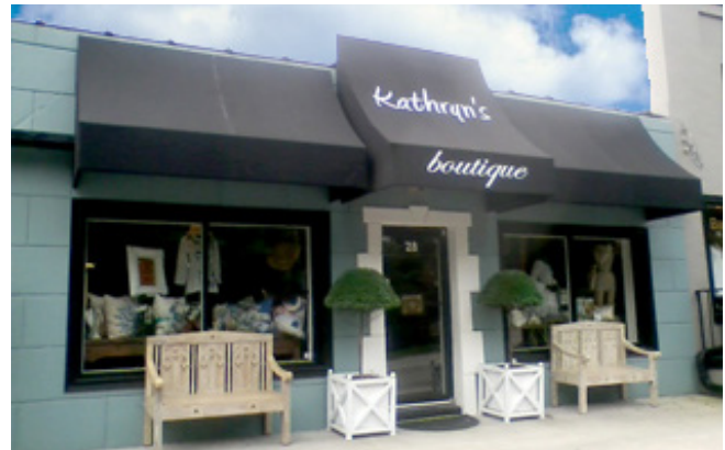
Canopy articulating main entry
