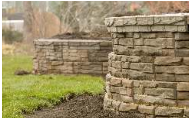
Example of stone wall
