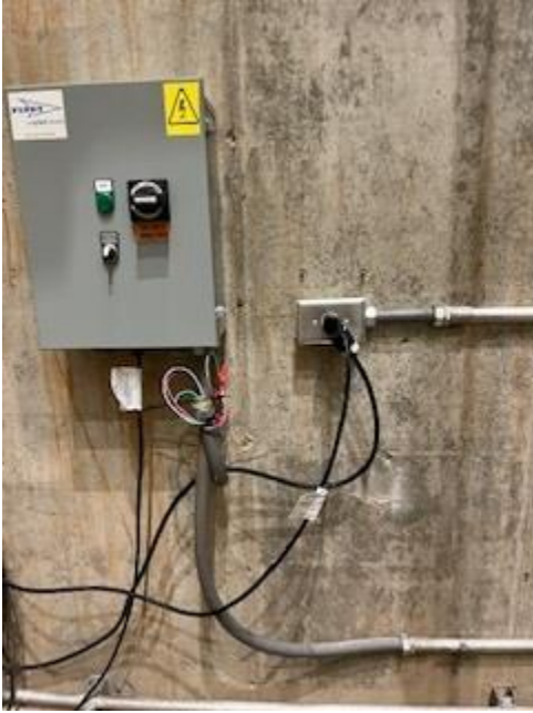
Installed out and New float for sump pump at Lake Keowee pump station.
