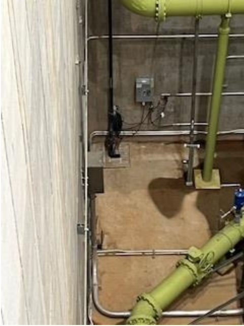
Installed out and New float for sump pump at Lake Keowee pump station.
