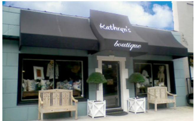
Canopy articulating main entry
