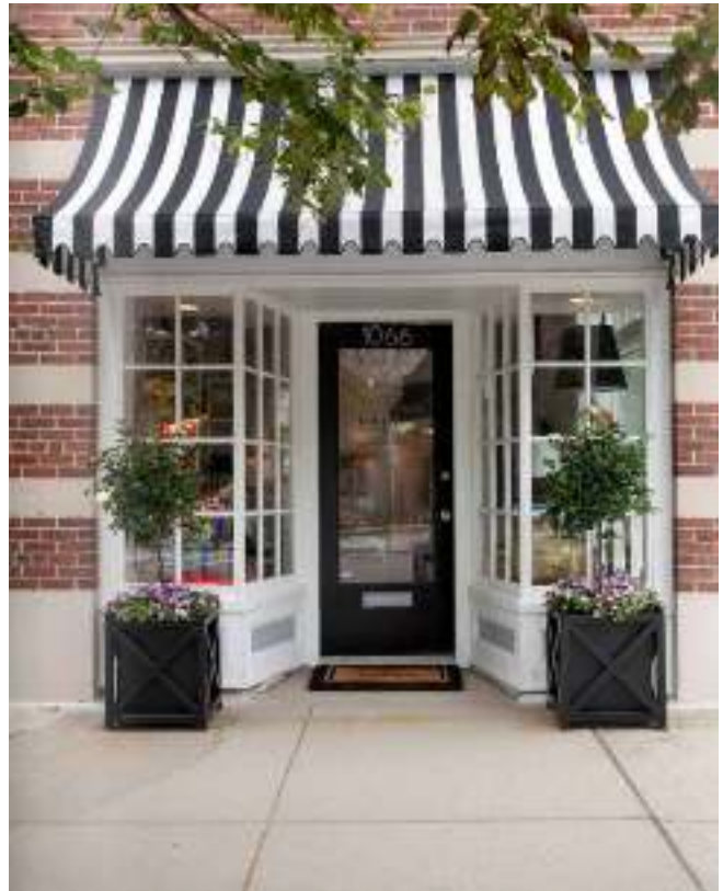
Example of primary entrance
