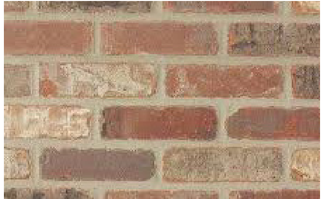
Masonry material example
