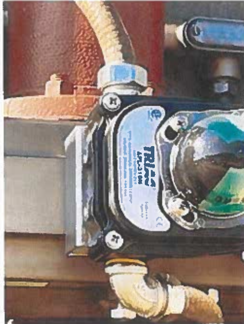
Replaced actuators on blow downs at the water plant.
